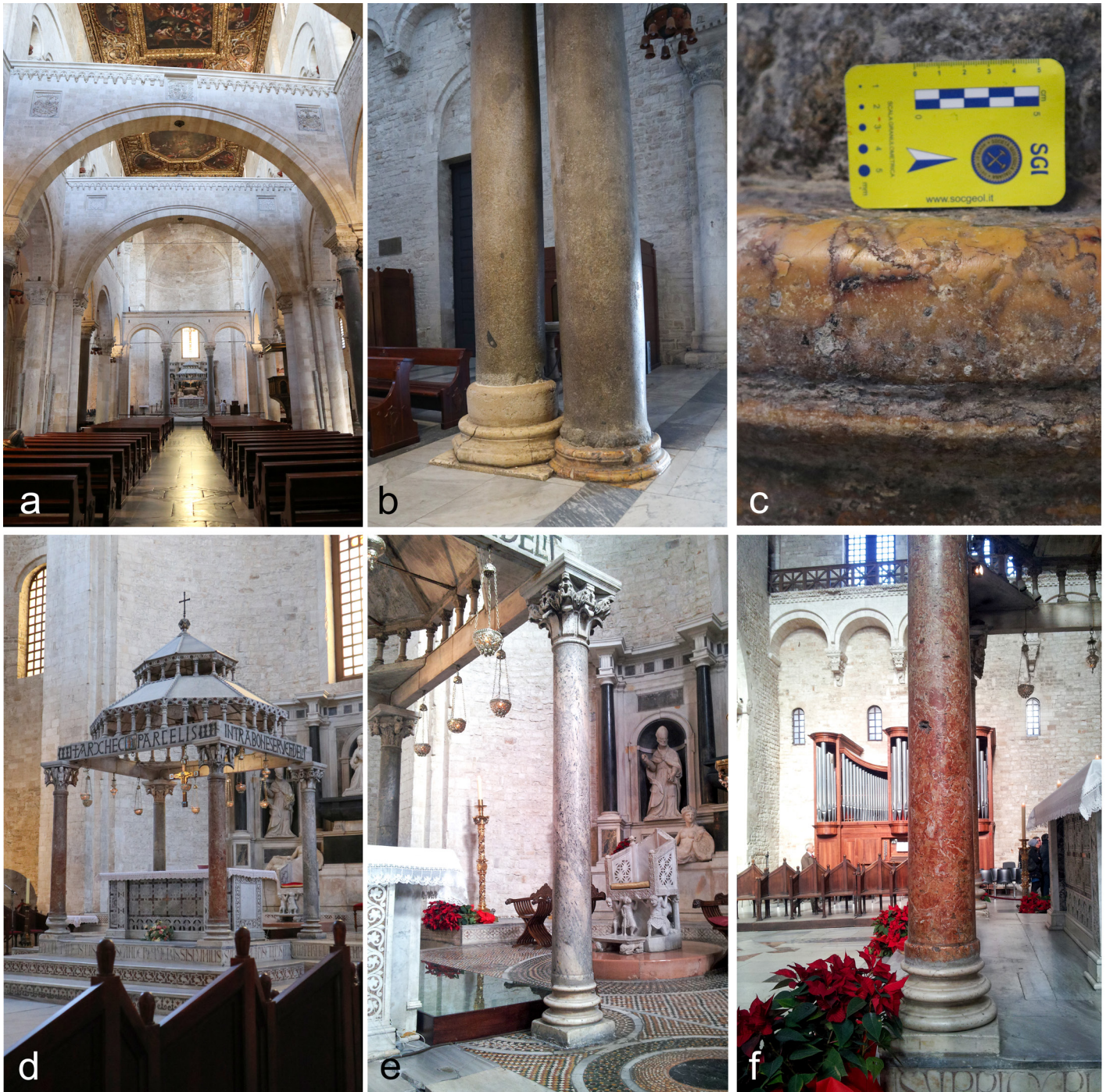
Fig. 9 - The central nave of the Basilica of St. Nicholas (a), two spolia columns in marmor troadense (b), a particular of a column basement in marmor numidicum (c), the ciborium (d) and a particular of the columns in greco scritto (e) and marmor triponticum (f).
