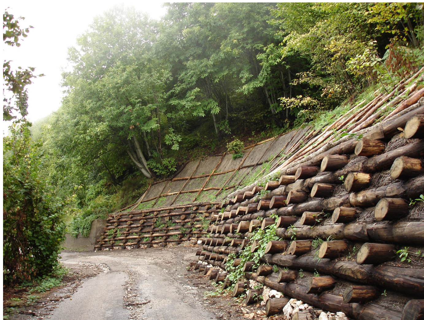
Fig. 18 - Soil bioengineering techniques (live cribwalls and blankets) at Vallone Castagnitiello (Sarno).
