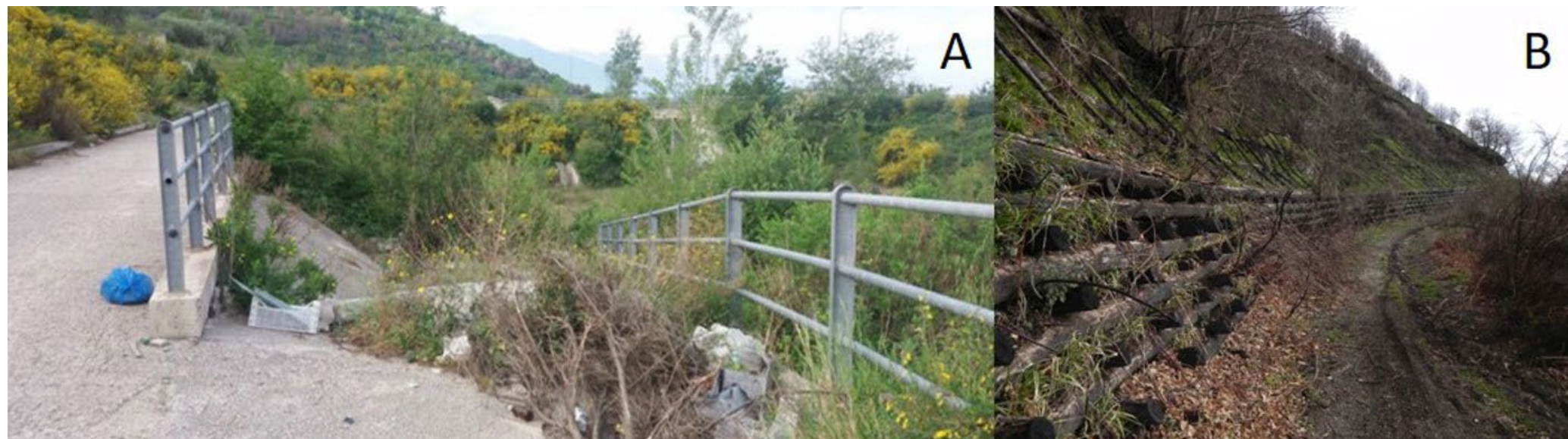
Fig. 19 - (A) Tree trunks and damp at San Vito retention basin ( www.sarnonotizie.it ) and (B) burnt live cribwalls (Sarno).
