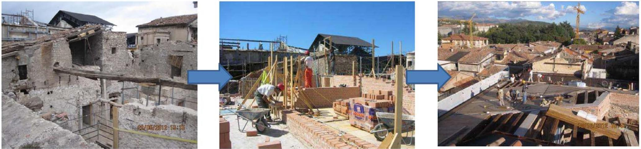
Fig. 77 - Reconstruction of the wooden roofs conserving the original configuration.
