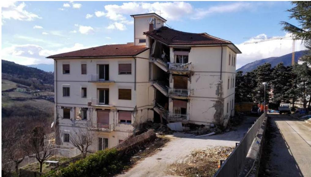
Fig. 63 - Example of RC building suffered severe damage in Via Cola dell'Amatrice during the April 6, 2009 main shock.
