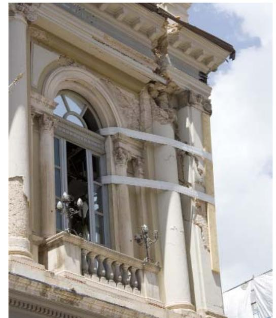
Fig. 71 - Particular of the Biblioteca Tommasi. The building was very severely damaged: the main facade was in danger of collapsing.
